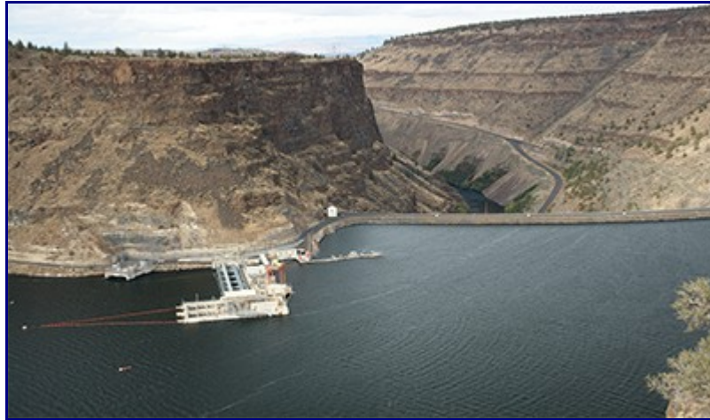
Round Butte Dam. Selective Water Withdrawal Tower and Fish Collection Facility is housed in the structure in the left of the photo. Photo by Greg McMillan.
